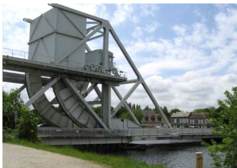
New Pegasus Bridge, Benouville
