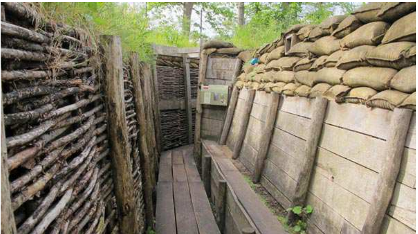
Trench with firing step.
