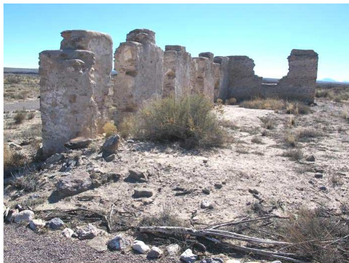
Fort Craig, what remains. Two walls of the commanding officer's quarters.
