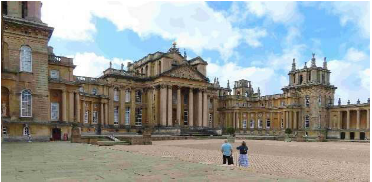
Blenheim Palace, front view
